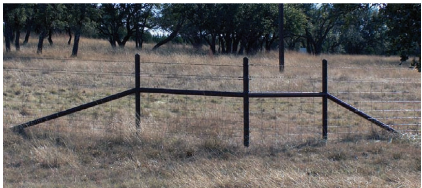
Permanent corner brace.
